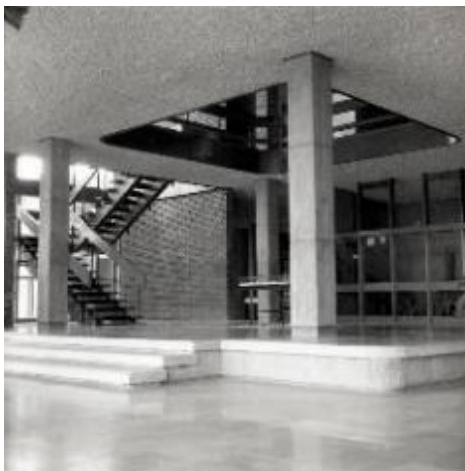
Figure 37 Two column types used in the Faculty of Architecture building: Square section columns in the gallery space of the Dean's Block (left) and rectangular section columns in the gallery space of the H block (right) (Models are produced by the Author, below photographs: Salt Archives)
