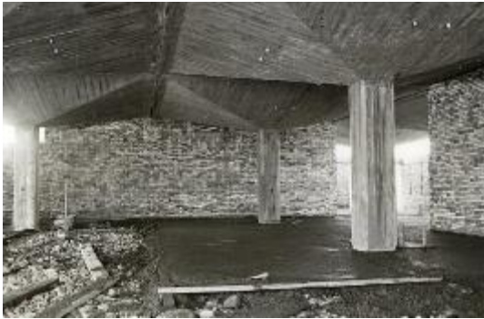
Figure 28 Similar exposed concrete pitched ceiling design of Çarşı Complex (left) and Cafeteria buildings (right). (Models are produced by the Author, photographs from METU Archives)
