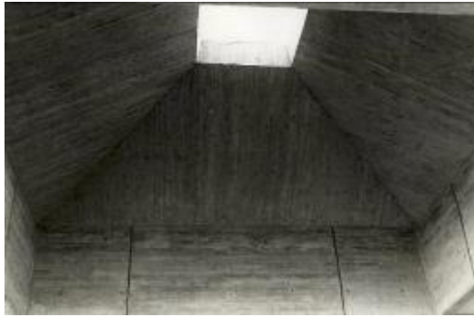
Figure 28 Similar exposed concrete pitched ceiling design of Çarşı Complex (left) and Cafeteria buildings (right). (Models are produced by the Author, photographs from METU Archives)
