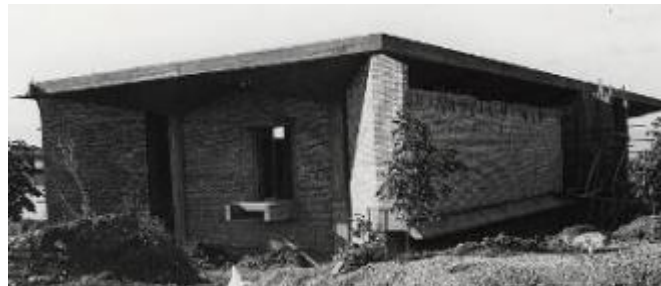
Figure 74 Şahniş designed for the Faculty of Architecture building: perspectival sketch and detail drawings by Çinicis. (above, Salt Archives) Exposed concrete şahniş on the West façade of Cafeteria building and glass şahniş located at the discotheque block of Çarşı Complex (below, METU Archives)
