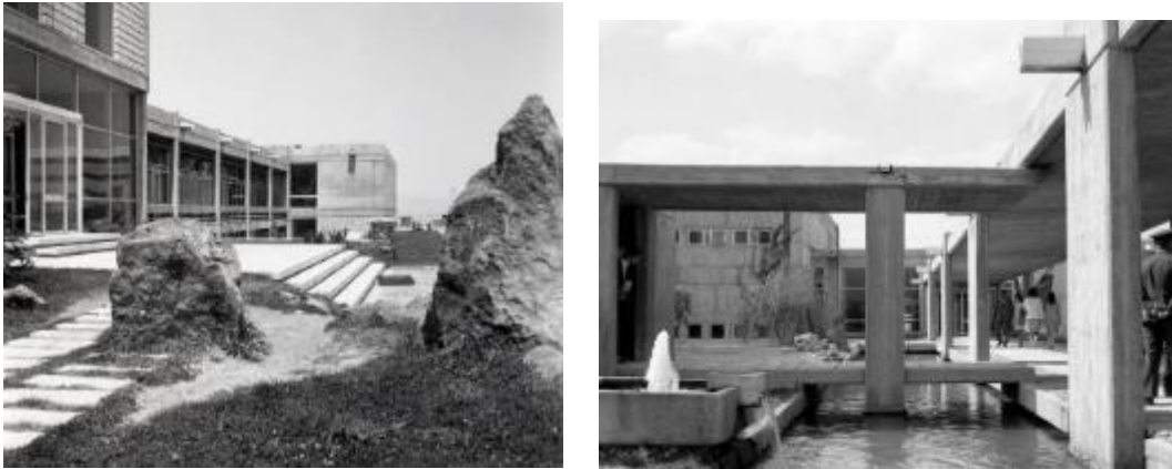
Figure 51 Two common use of water spouts at the Faculty of Architecture building which are modeled to be included in the Archive Box; water spouts in front of the balcony that circulates rain-water into independent white exposed concrete water bowls with the help of metal chains to control draining route of the water (left) and rectangular water-spouts extends from the arcade eave at the main entrance fall rain-water into the pool. (right) (Salt Archives)
