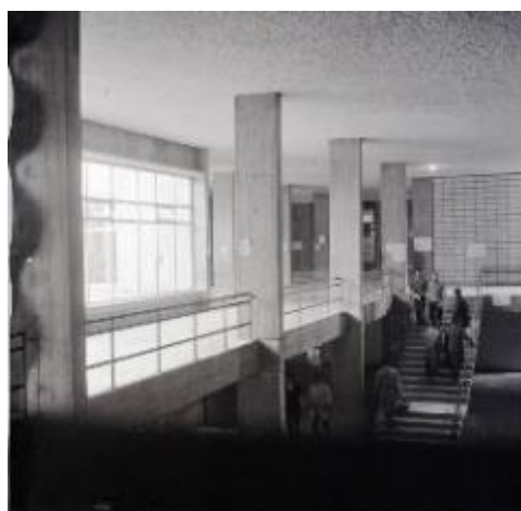
Figure 37 Two column types used in the Faculty of Architecture building: Square section columns in the gallery space of the Dean's Block (left) and rectangular section columns in the gallery space of the H block (right) (Models are produced by the Author, below photographs: Salt Archives)
