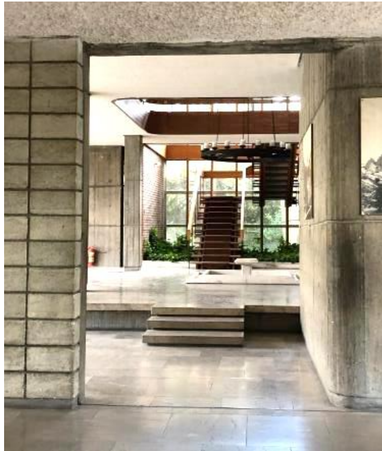
Figure 68 Photograph of the Dean's Block documents decorative elements including metal circular chandelier, marble fountain, hornbeam balustrade with curved corners, beton-brut columns and landscape arrangement under wooden staircase in the gallery space. (Photograph by Tunahan Çalışır)
