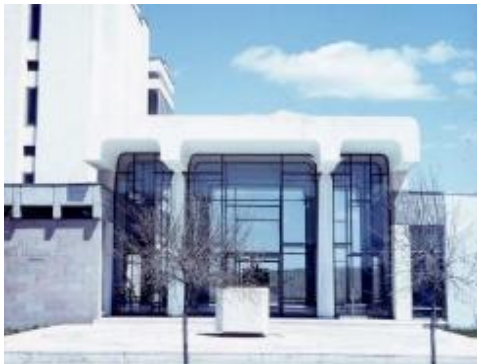
Figure 38 Reproduction of columns located in the Library building (left) and the School of Mathematics building (right) (Produced by the Author) Exposed white concrete columns with capitals carry entrance eave roof of the library building and exposed concrete columns with capitals carry the arcade eave of the School of Mathematics. (left photograph: Salt Archives, right: METU Archives)
