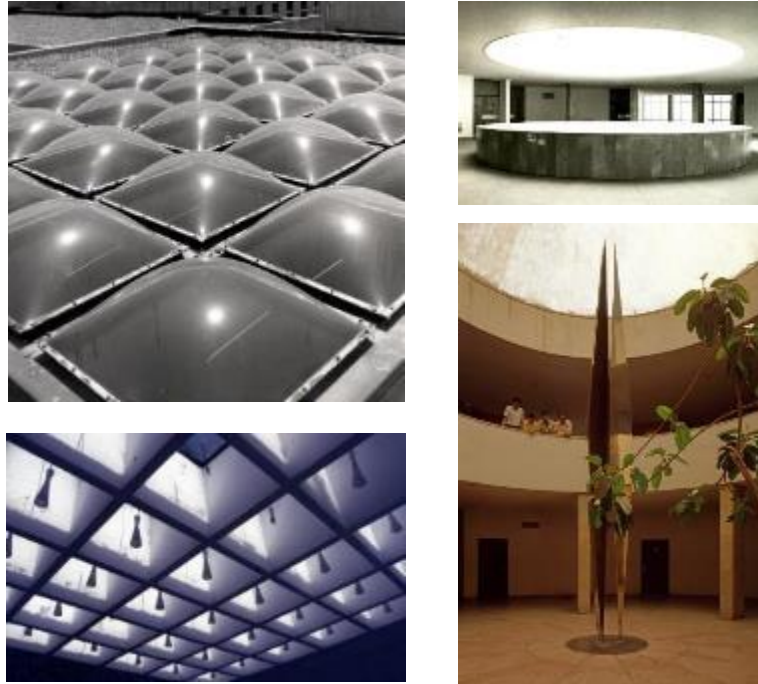
Figure 19 Photographs of the skylights in Faculty of Architecture from interior and roof. (left, Salt Archives) & Photographs of the gallery space in Physics auditorium block from ground and basement floors. Space is highlighted with transparent polyester dome and abstract sculpture (1968) by the artist Şadi Çalık.. (right, Salt Archives)
