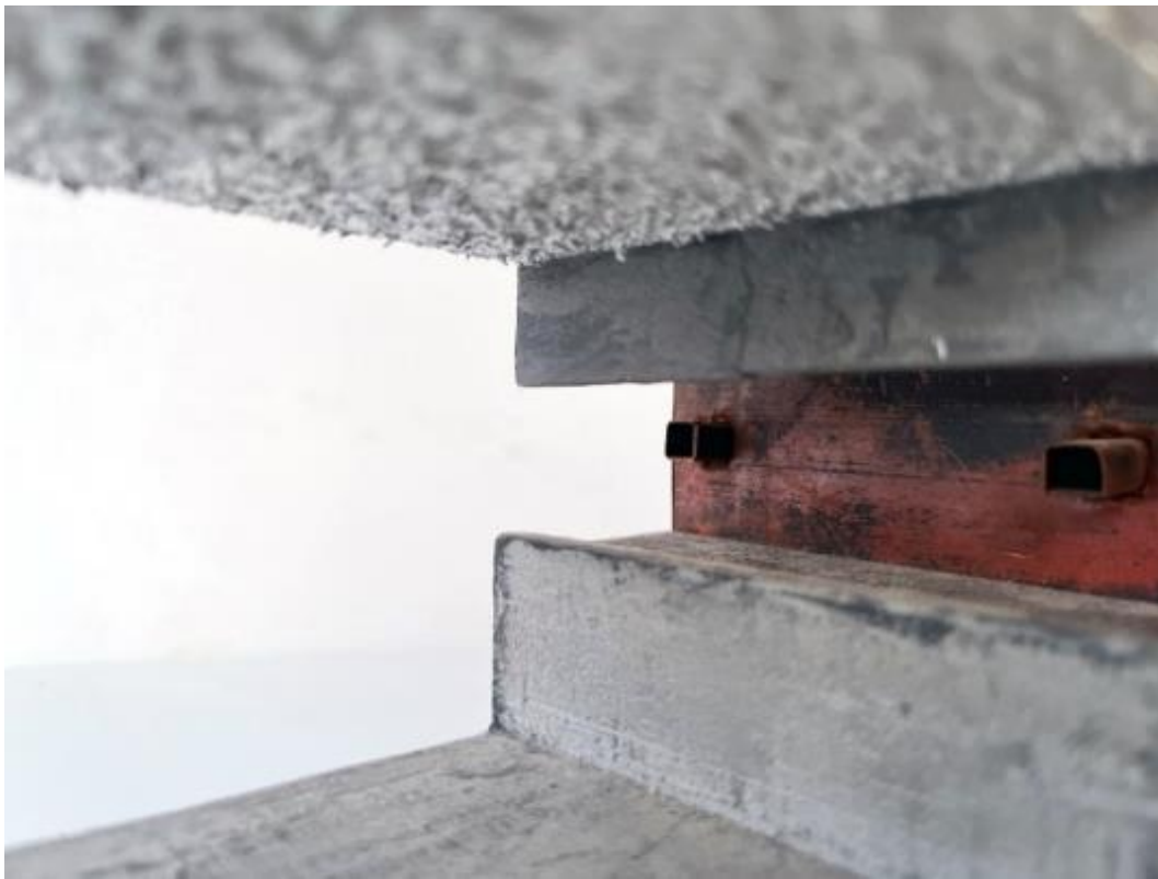
Figure 52 Illustration of white exposed concrete water spout extends from the facade of the inner courtyard (above) and water spouts made out of Ankara stone attached to the walls retaining upper soil of the inner courtyard at the Faculty of Architecture building. (Produced by the Author)
