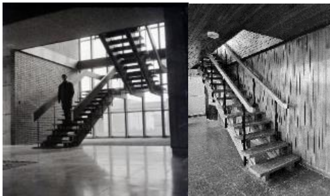
Figure 31 Illustration of staircase at Deans' Block. (above, produced by the Author) Below: Timber staircase at Dean's block (left, Salt Archives) also re-utilized for the museum block (right, photograph by the Author).
