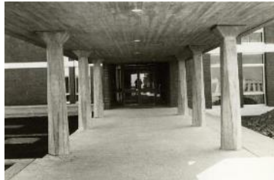
Figure 38 Reproduction of columns located in the Library building (left) and the School of Mathematics building (right) (Produced by the Author) Exposed white concrete columns with capitals carry entrance eave roof of the library building and exposed concrete columns with capitals carry the arcade eave of the School of Mathematics. (left photograph: Salt Archives, right: METU Archives)
