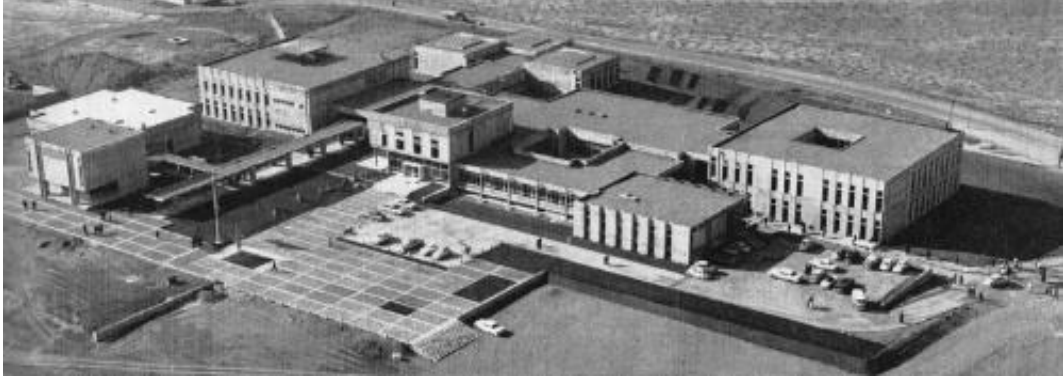
Figure 1 Areal photograph of the Faculty of Architecture Building Complex. (Salt Archives)
