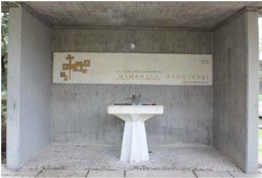
Figure 11 U shaped walls at the Faculty of Architecture building. (Produced by the Author.)
